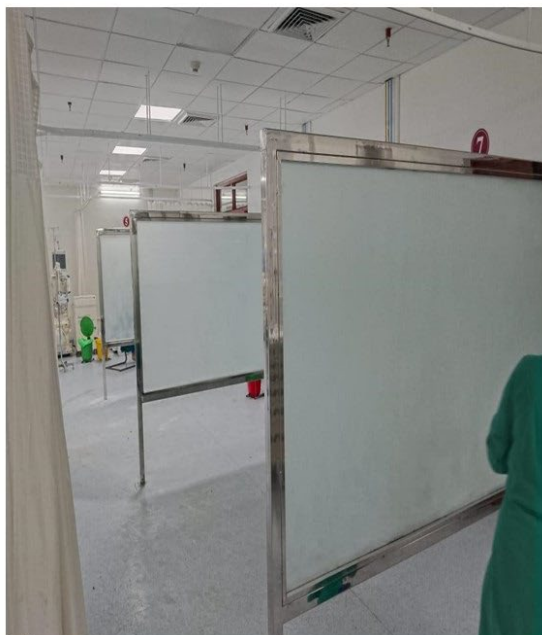
5. Providing & fixing toughened frosted glass wall partition with steel frame between all beds in AICU, D&T-OT third floor at AIIMS, Jodhpur.jpg
