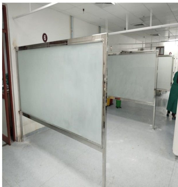
5. Providing & fixing toughened frosted glass wall partition with steel frame between all beds in AICU, D&T-OT third floor at AIIMS, Jodhpur.jpg
